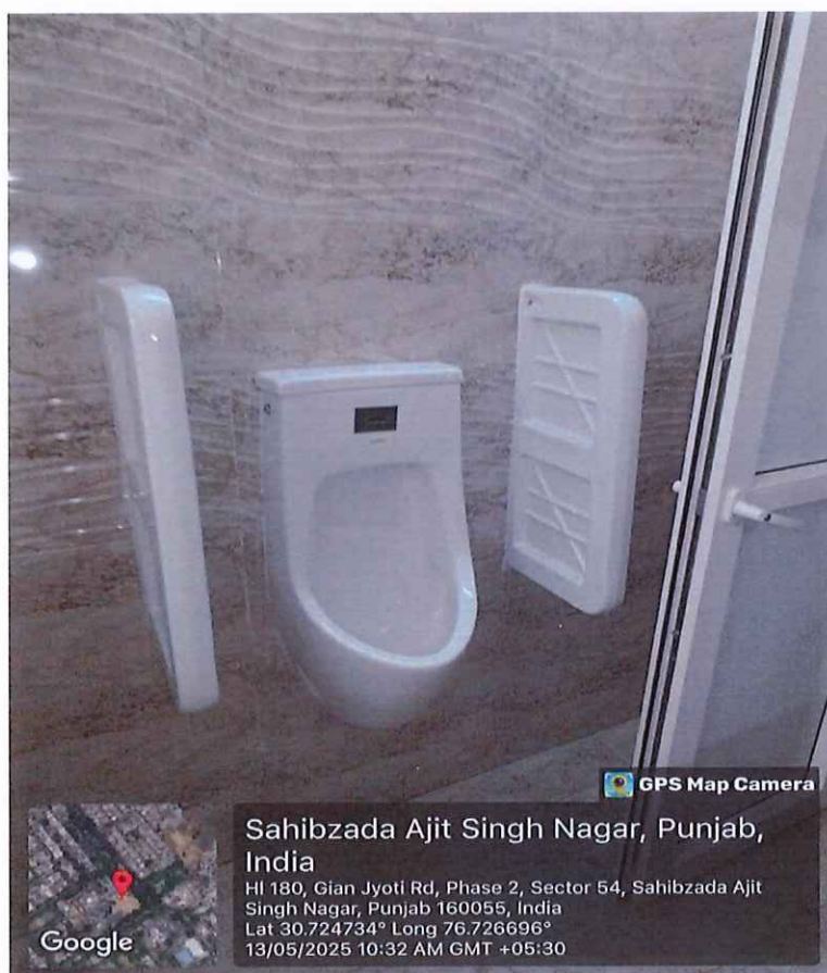
Urinal Sensor Flusher installed in Washroom
