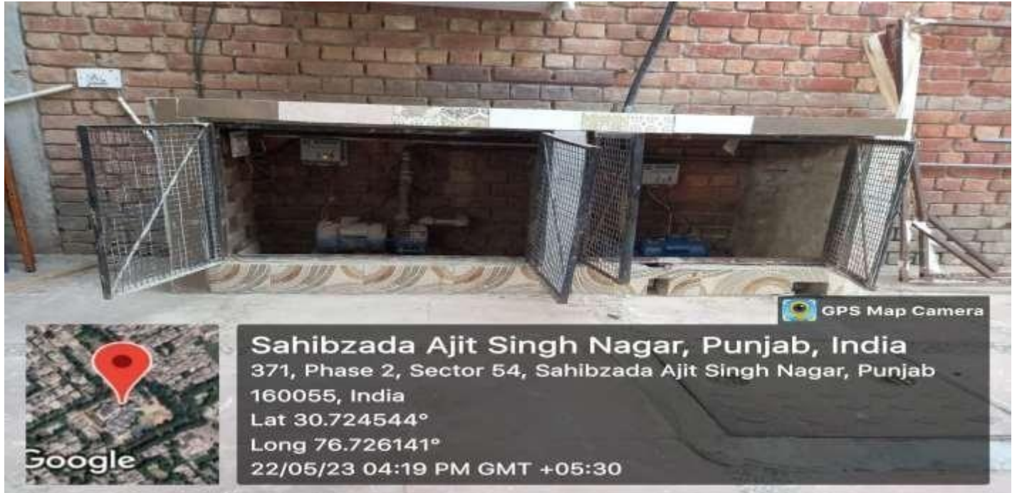
Motor – Pump sets transporting water from underground tanks to overhead water tanks
