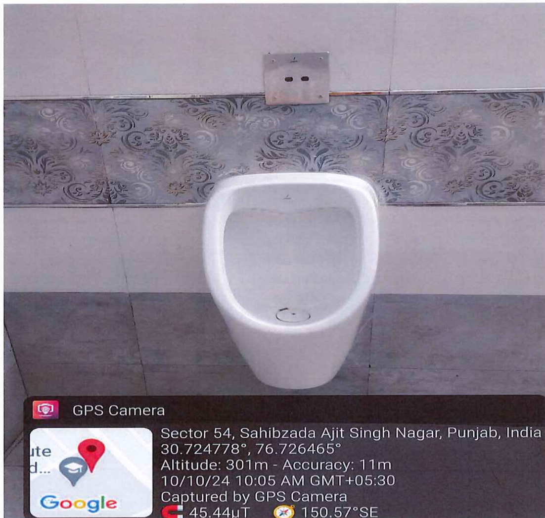
Automatic Sensor urinal for differently -abled
